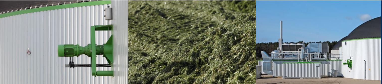
The digester, with its powerful and robust agitator, forms the core of every biogas plant. The continuously operating REMEX® agitator is designed for the mixing of energy crops and slurry in the first- and second-stage digesters of the biogas plant.
